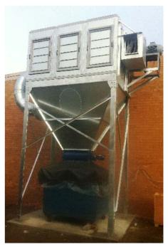
The units are supplied standard with a Rotary (airlock) Valve that feeds the collected waste from the Dust Collectors Hopper directly into a 3m³ waste bin. The waste bin can be emptied without the Dust Collector being turned off by simply turning off the Rotary Valve. This eliminates the need for stopping production in the factory. This equated to big savings in labour costs. All Units are available with a energy saving VSD as an option
