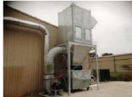
The unit is also supplied with a Polex Variable speed Drive Controller or VSD. The VSD is supplied with a pressure transducer that will sense and automatically turn the power consumption of the fan motor down when one or more of the machines is not in use. **This equates to big savings on power consumption**. Lambert Kitchens is very happy with the performance of the unit, the ducting & the service they received from Ezi-Duct and Polex Environmental Engineering.
