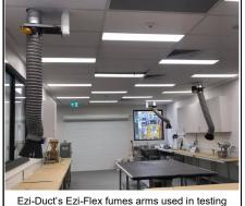
The hood is manufactured from robust light weight steel construction and is fitted with an aluminium handle making the EziArm very light & manoeuvrable. The client is delighted with the simple operation of the EziArm Telescopic Fume Arms in keeping the fine dust away from the lab technicians.
