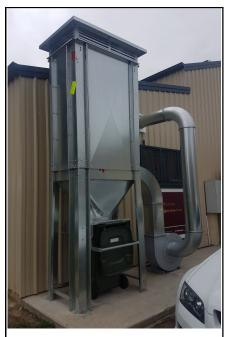
Econo 4000 WB installed outdoors. Wheelie bin option makes dust removal easy.
