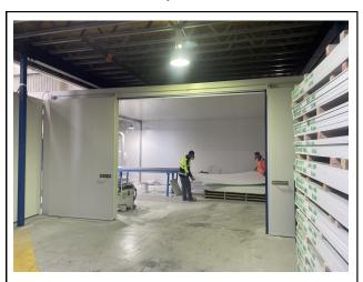
Specially designed room to contain the concrete dust
