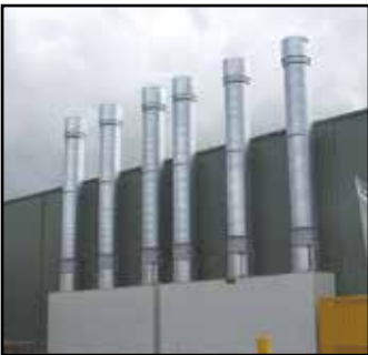
Stacks with Axial flow fans & weather cowls flap type
