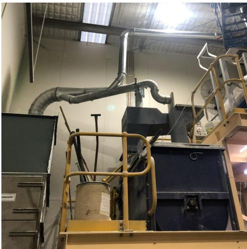
Ezi-Duct's NSW team has just finished making modifications to an existing dust collection system for a western Sydney factory that specializes in gardening supplies. We used our modular ducting to make modifications to the existing ducting system in order to deal with the chemical dusts that is created during the filling process.
