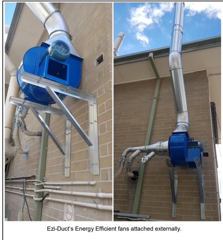
Ezi-Duct's Energy Efficient fans attached externally.
