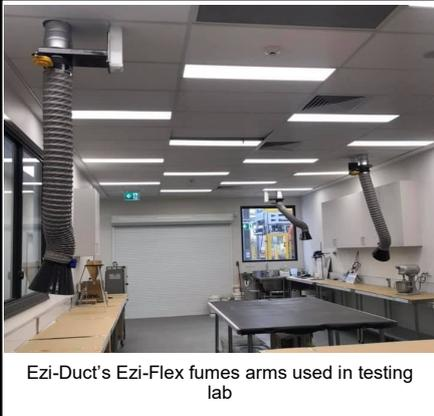
Ezi-Duct's Ezi-Flex fumes arms used in testing lab
