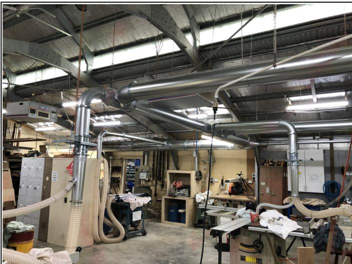
*Ezi-Duct modular ducting system installed at the men's shed.*
