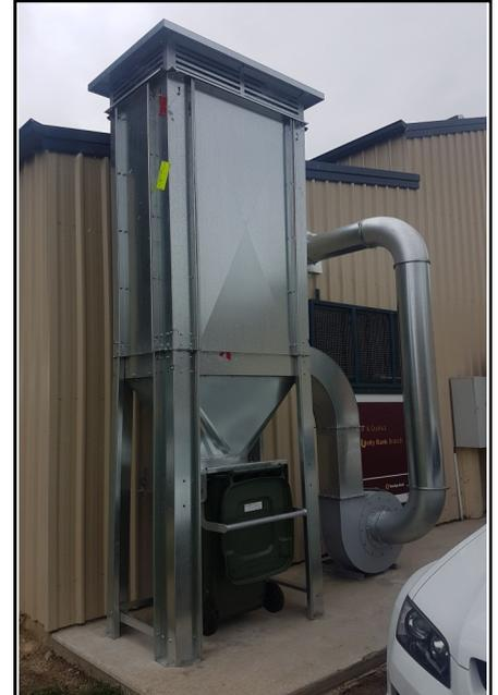
*Econo 4000 WB installed outdoors. Wheelie bin option makes dust removal easy.*
