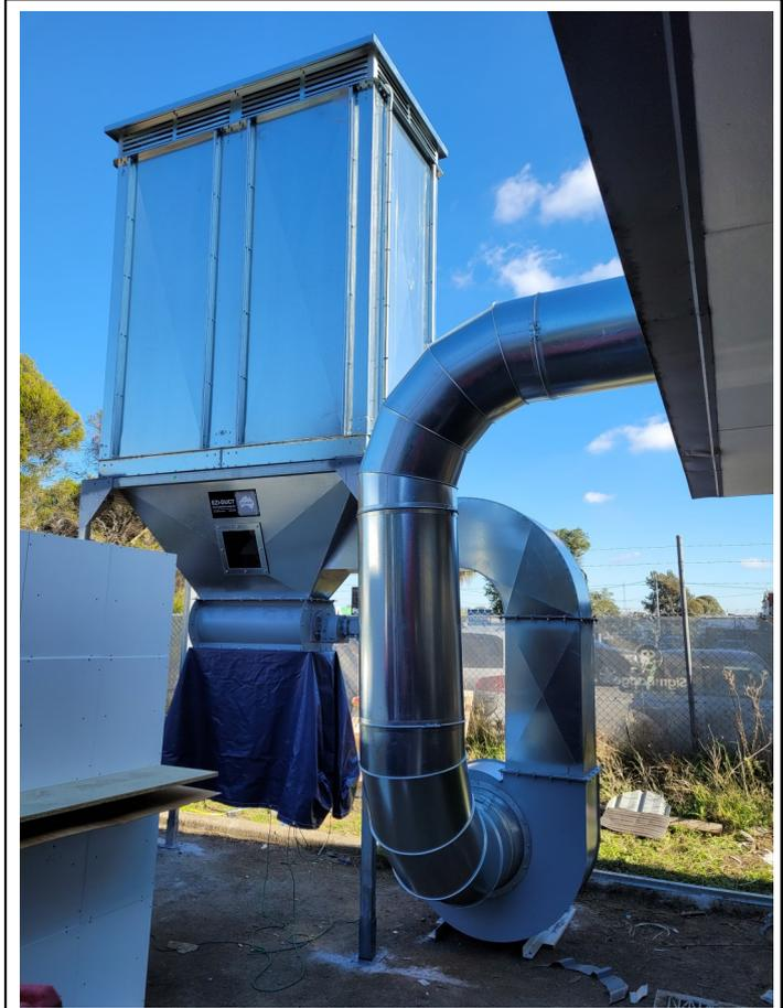
ECONO 15000 HRV installed, all the waste will drop directly into a giant bin.
