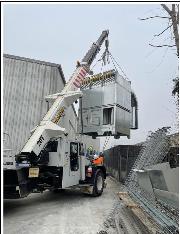
Crane lifting the MDC body into location
