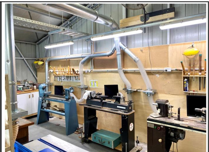
Ezi-Duct's modular ducting was run throughout the workshop and connected with our flexible ducting.
