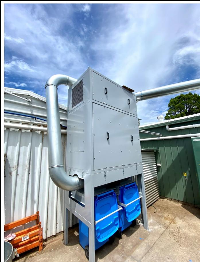
ECompact 12000WB installed, all the waste will drop directly into a giant bin.
